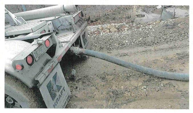
Picture 5: Pneumatic Tanker Connected to Mixing Hopper - Ready to Unload
