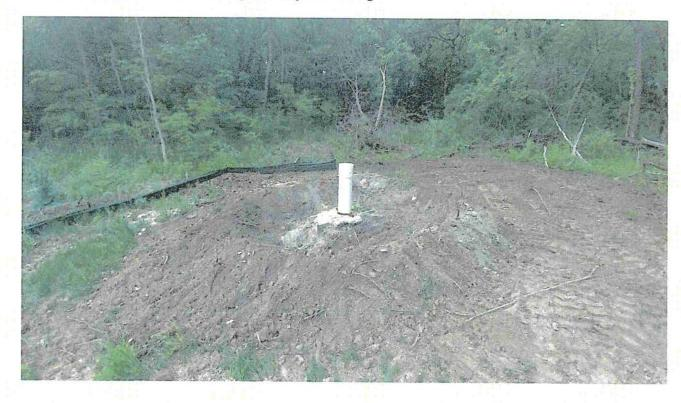
Picture 3: Custom Mixing Hopper on Injection Casing with Containment Berm
