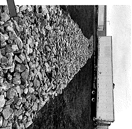
Rocked drainage ditch from trailer lot to cow pasture and OF 008
