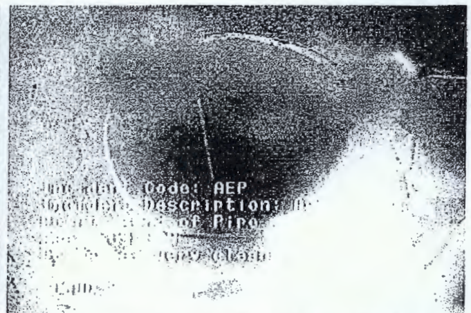
AEP - Access Point - End of Pipe @ 300.9 ft. very clean
