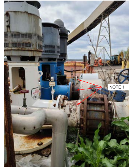
CDS PUMPS DISCHARGE HEADER. PHOTO TAKEN LOOKING SOUTHEAST. SCALE: NTS 1 THIS SHEET
