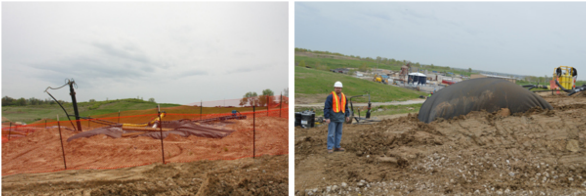
Photos of reinforced concrete pipes (left SC-2 and right SC-4) covered in flexible membrane liner before abandonment. SC-4 is under pressure from landfill gas.
