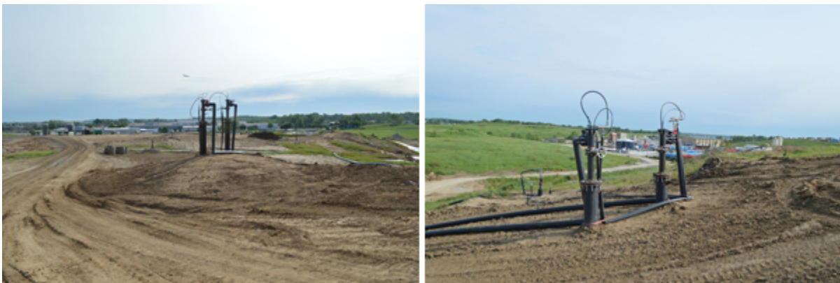
Photos of reinforced concrete pipes (left SC-2 and right SC-4) after abandonment.
