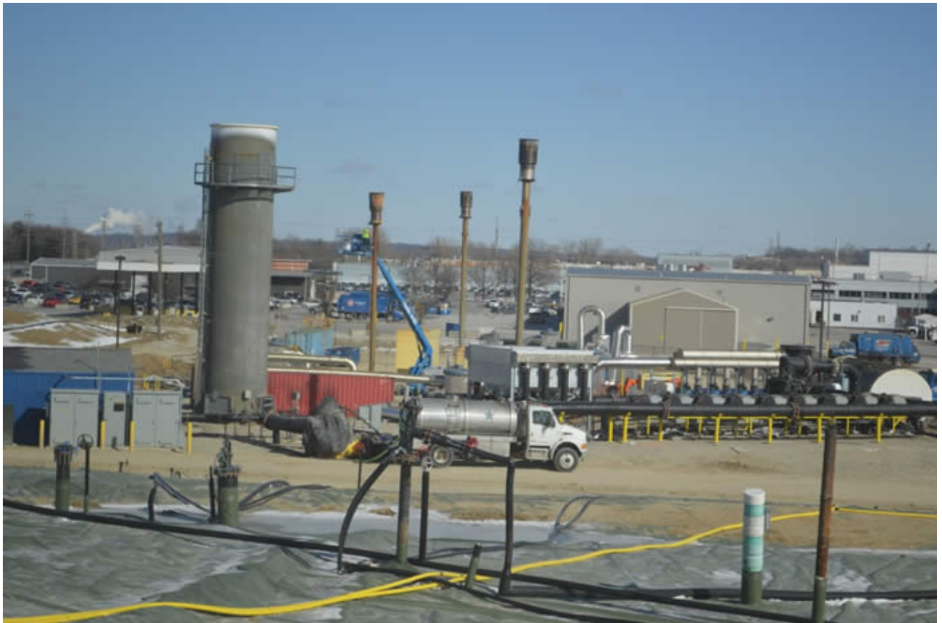
Photo of repair being made to flare at Bridgeton Landfill, Jan. 23, 2014.
