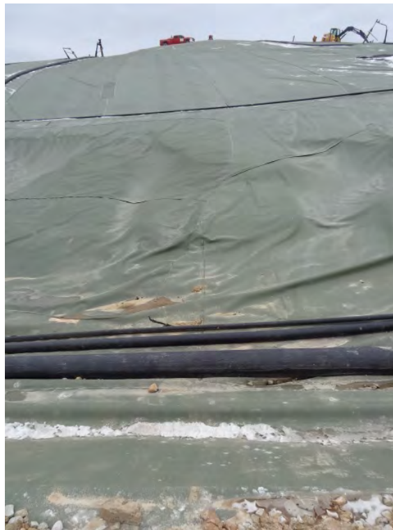
Figure 9. Photograph along south slope of south quarry showing slope collapse and/or slope movement features.
