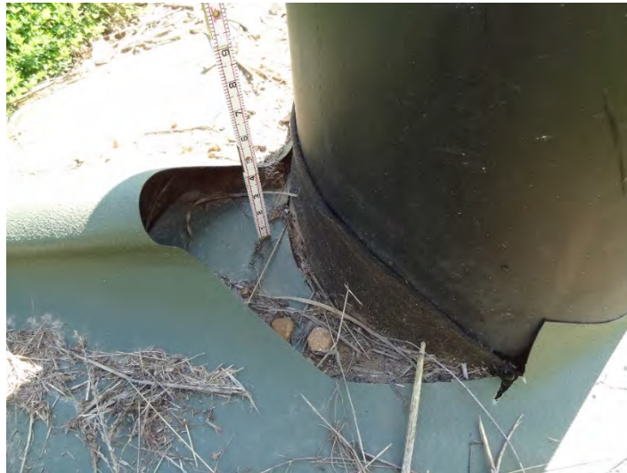
Figure 10. Photograph of geosynthetics around PS-35 not sealed to piping near maintenance building on northwest side of north quarry.
