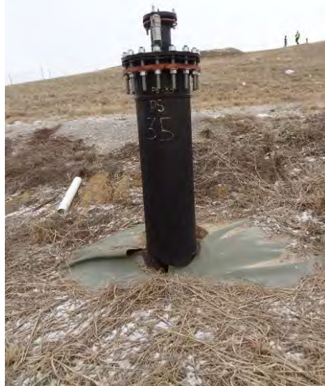
Figure 3. Photograph of geosynthetics around PS-35 not sealed to piping near maintenance building on northwest side of north quarry.
