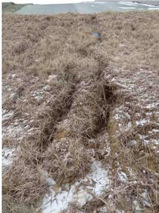
Figure 1. Photograph of erosion of the soil cover near the maintenance building on northwest side of north quarry.
