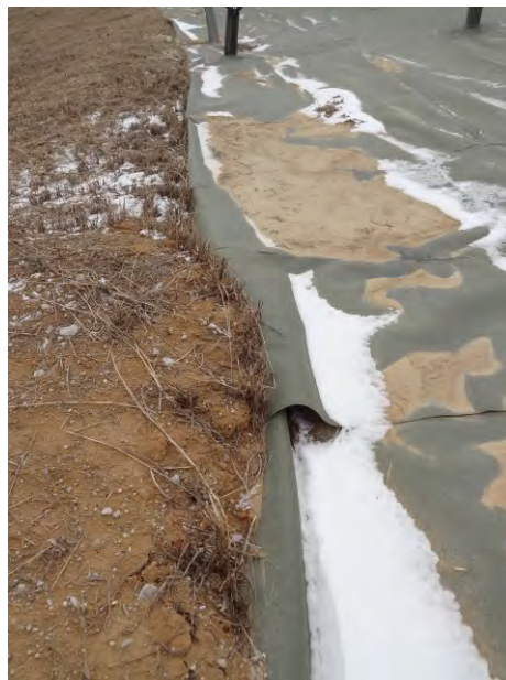
Figure 8. Photograph of unwelded geomembrane on northeast side of the north quarry near large flare station.
