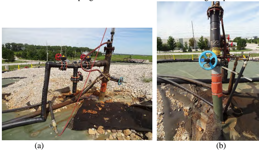
Figure 4. Photographs along south slope of south quarry showing remnants of leachate outbreaks.
