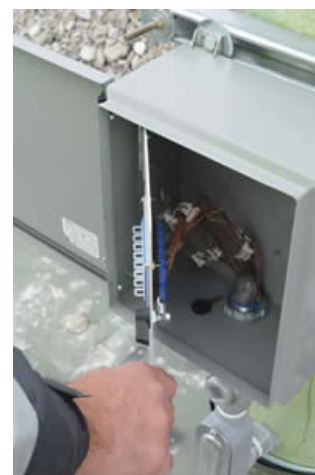
Photo of new temperature monitoring probe controllers installed in Nov. 2013 at Bridgeton Landfill.
