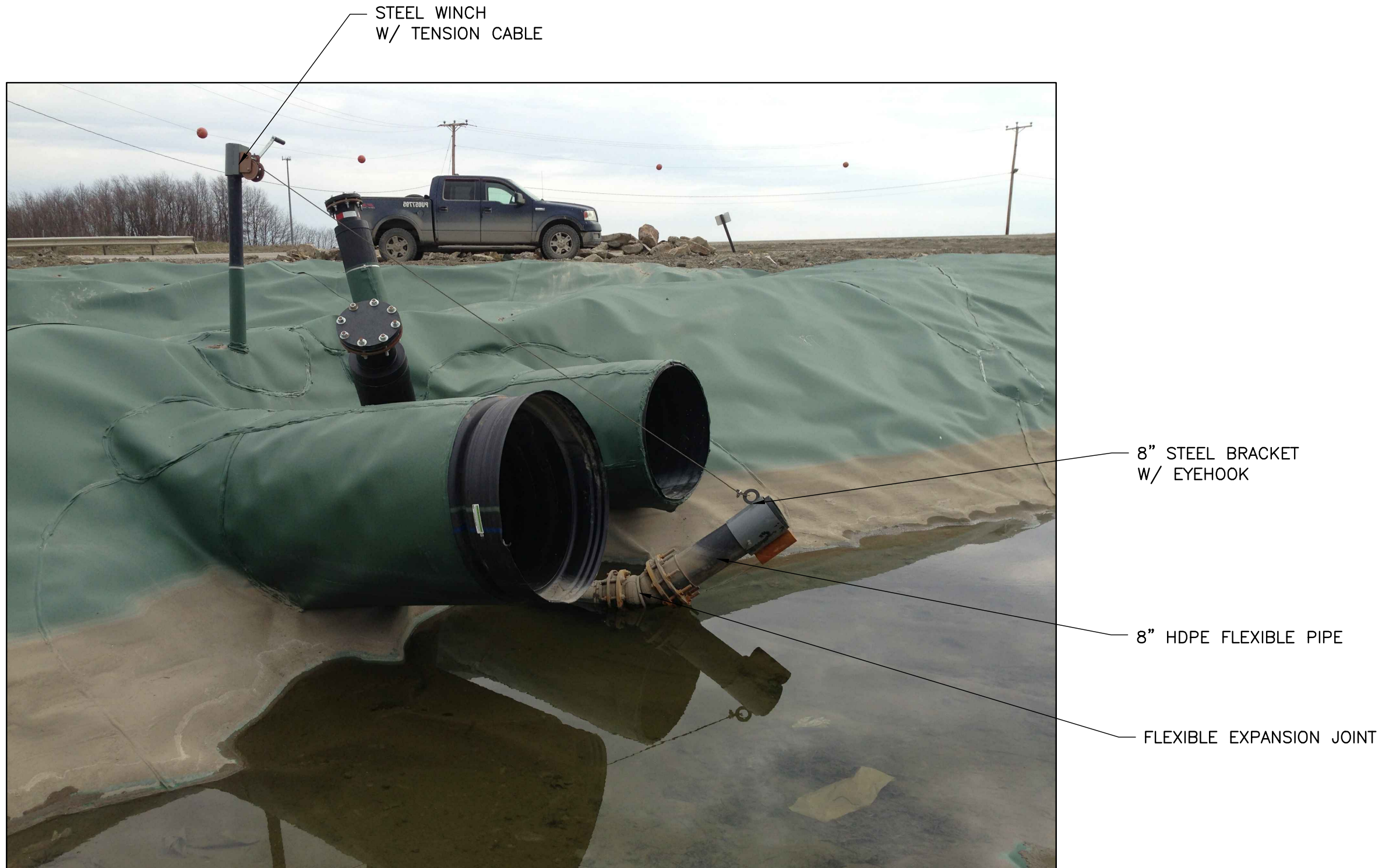
HDPE FLEXIBLE PIPE FOR ACCESS ROAD CHANNEL CROSSING
