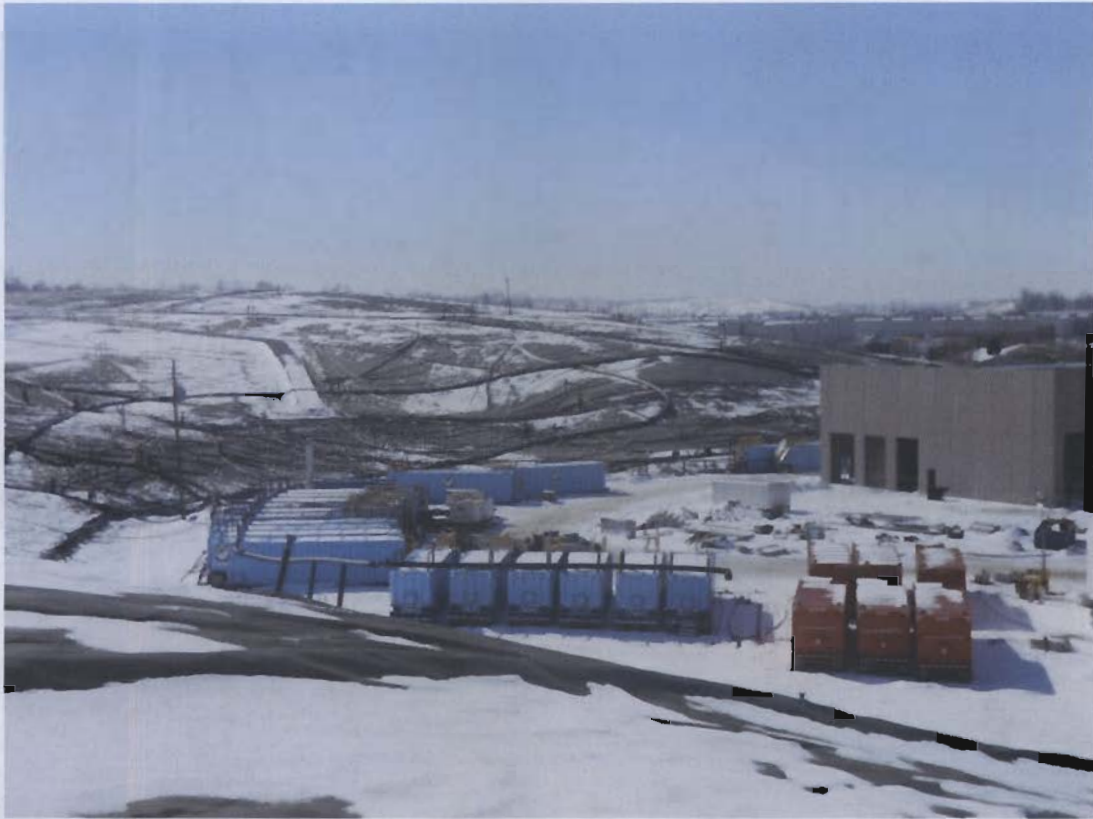
21. Tank Battery area (TB1-TB4); 6 emergency storage tanks on right.
