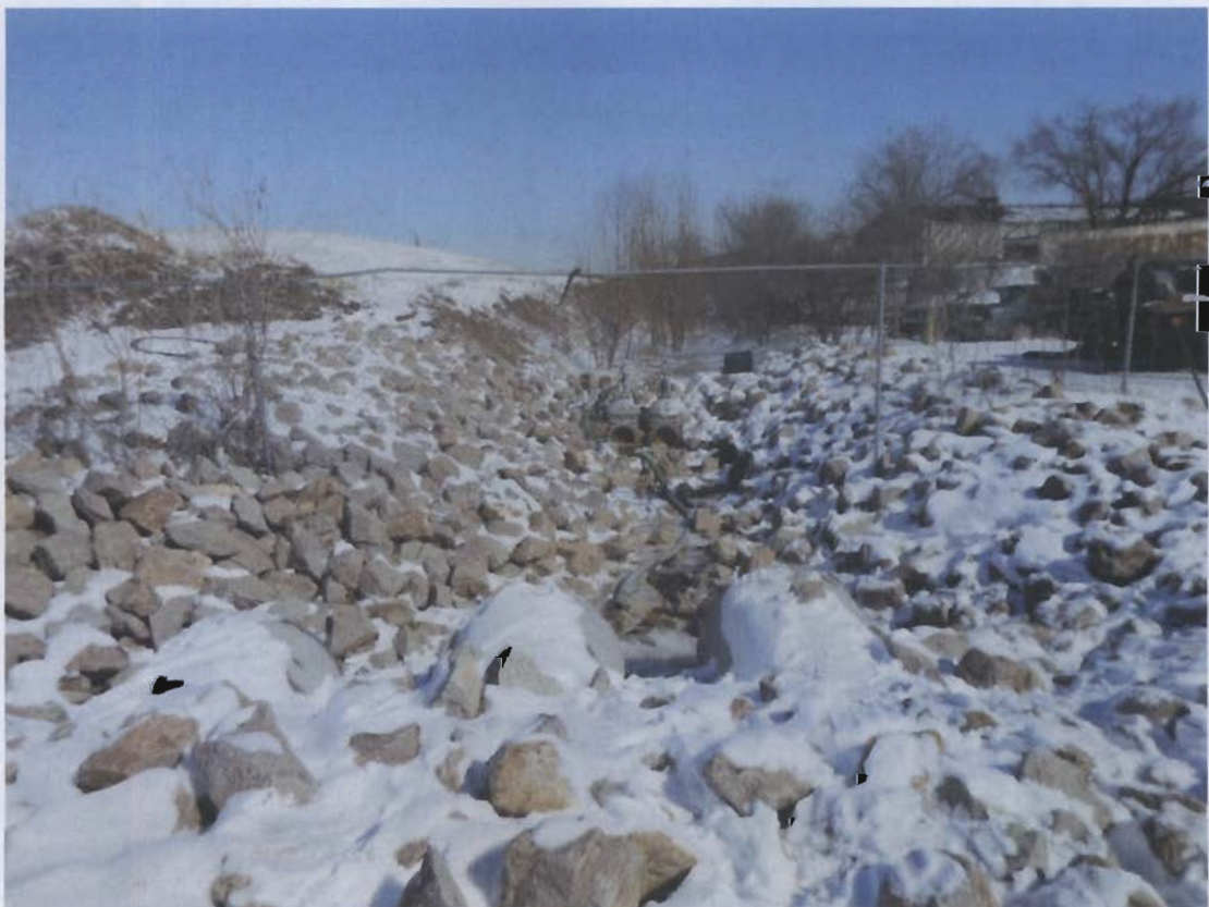
30. Outfall 003 (looking NE toward landfill).
