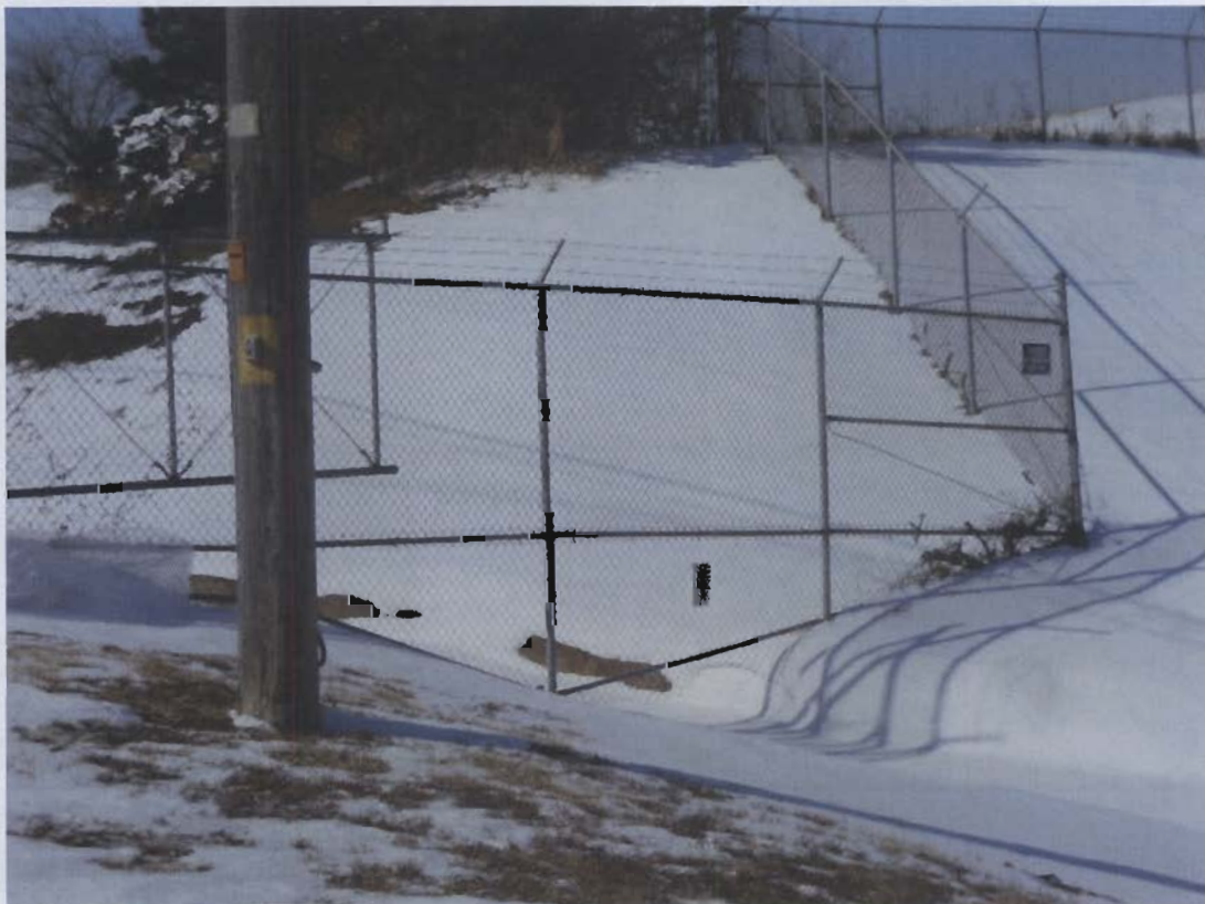
28. Outfall 007 (located along west side of entrance road).
