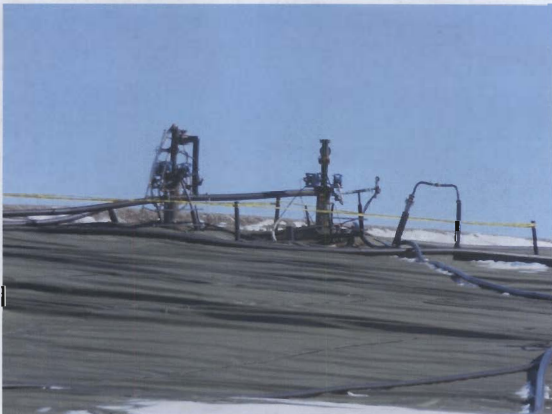
4. Subsided area #4 located at SC-5.
