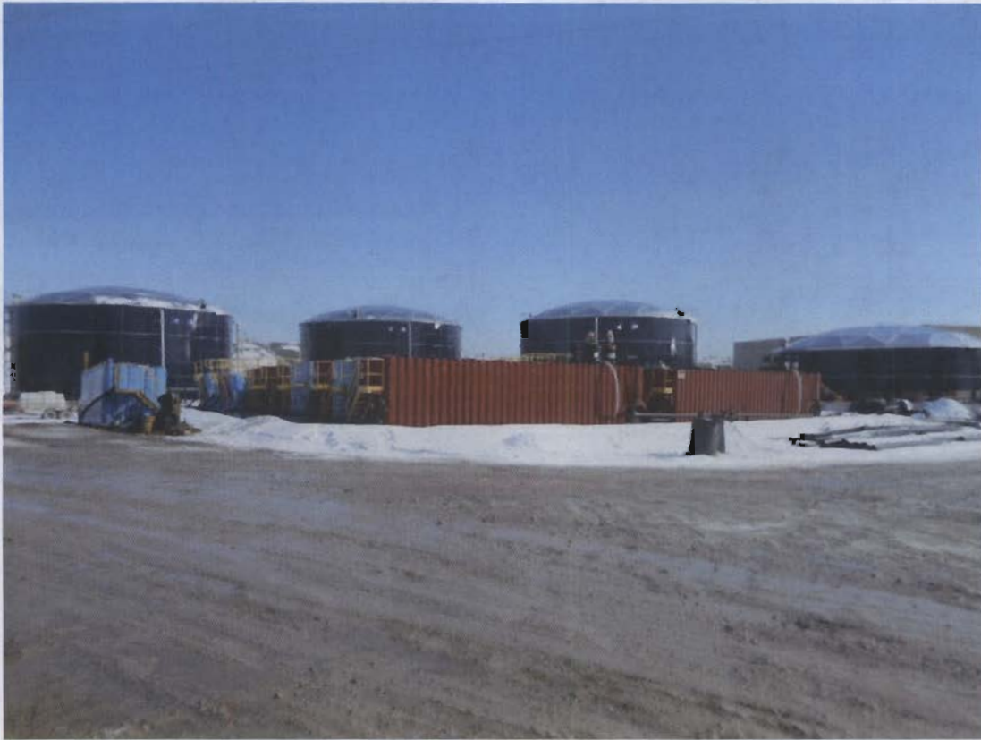
19. Buffer frac tank farm (24x); 1-M gallon tanks in background.
