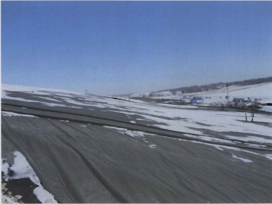
27. Southeast slope of landfill (looking NE).
