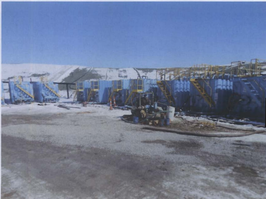
22. Truck load-out station at Tank Battery area.
