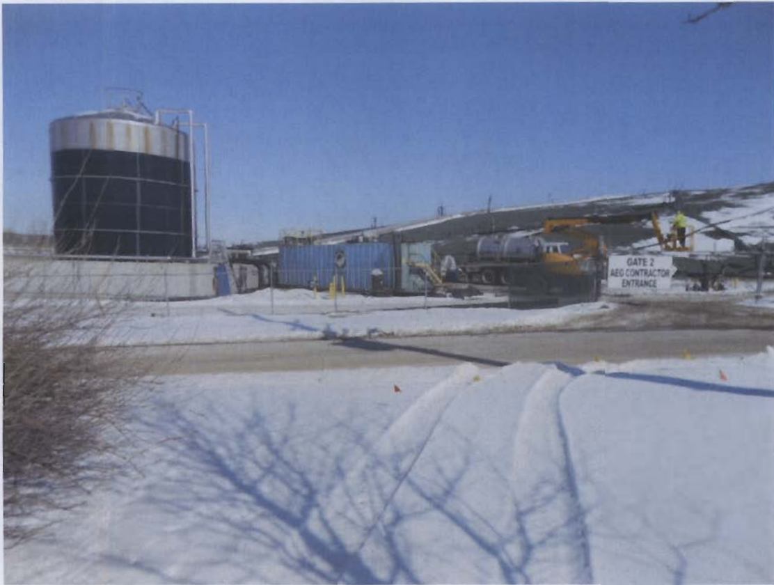
17. Frac tank at SW corner of landfill and 96K tank.
