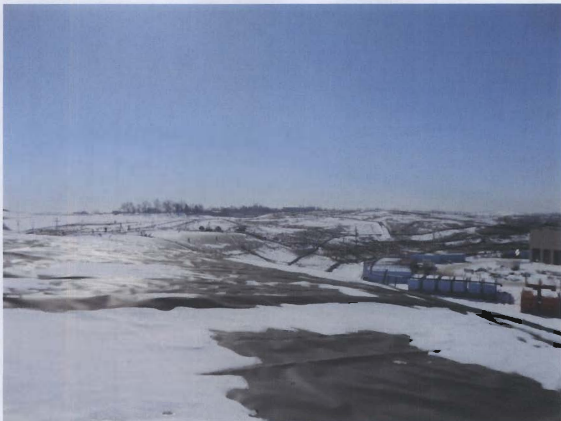
26. Overview of south quarry (looking south from north quarry).
