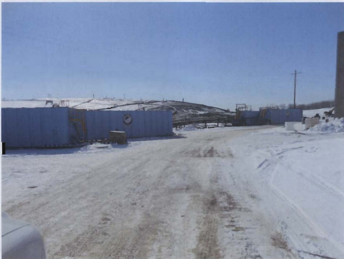
16. Frac tanks located in Amphitheater area.
