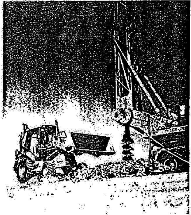
SCS professionals conduct field and laboratory testing to access LFG quantities, characteristics, current and future production rates, and optimal recovery system configurations.
