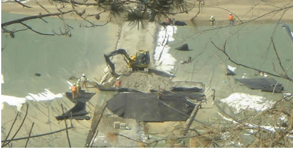
Photo of repairs being made to GEW-30R Bridgeton Landfill, Mar. 4, 2014
