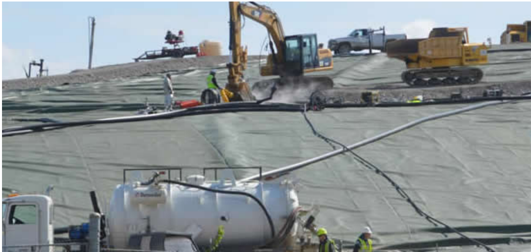
Photo of work on gas extraction well (GEW-21) on the south slope of Bridgeton Landfill, May 16, 2014
