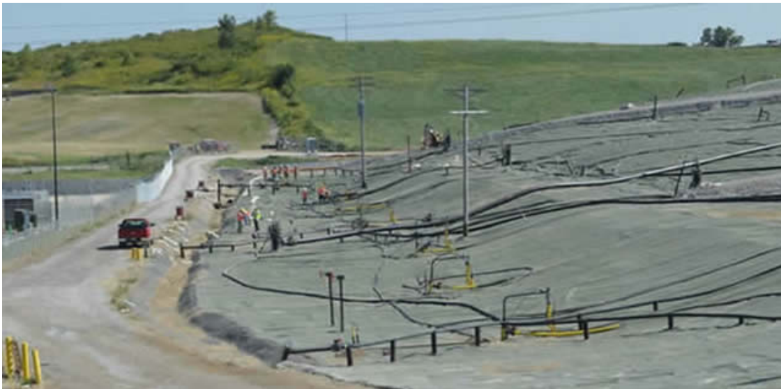
Photo of additional EVOH capping material installation.
