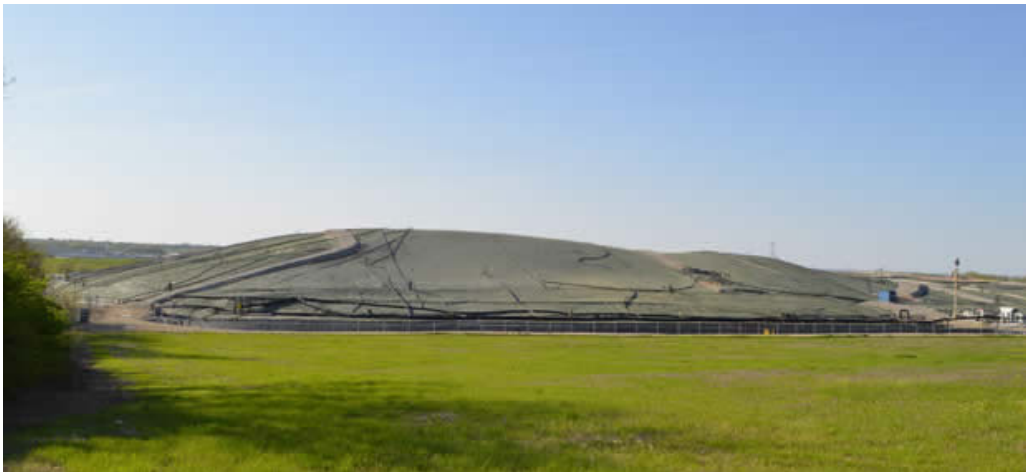
Photo of the South Quarry - Bridgeton Landfill, Apr. 24, 2014
