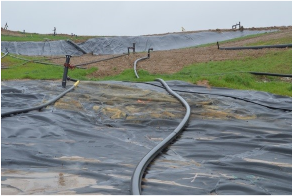
Photo 2. Heat deterioration of flexible membrane liner (FML), measured temp. 128°F, April 2013 (Source: MDNR Staff, 2013).
