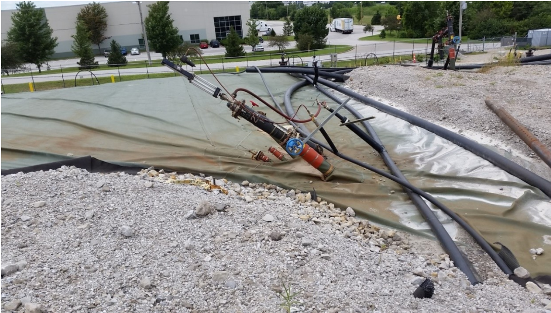
Photo11. Damaged landfill gas extraction infrastructure from the smoldering/heating event at BSL dated July 22, 2015 (Source: Todd Thalhamer 2015)
