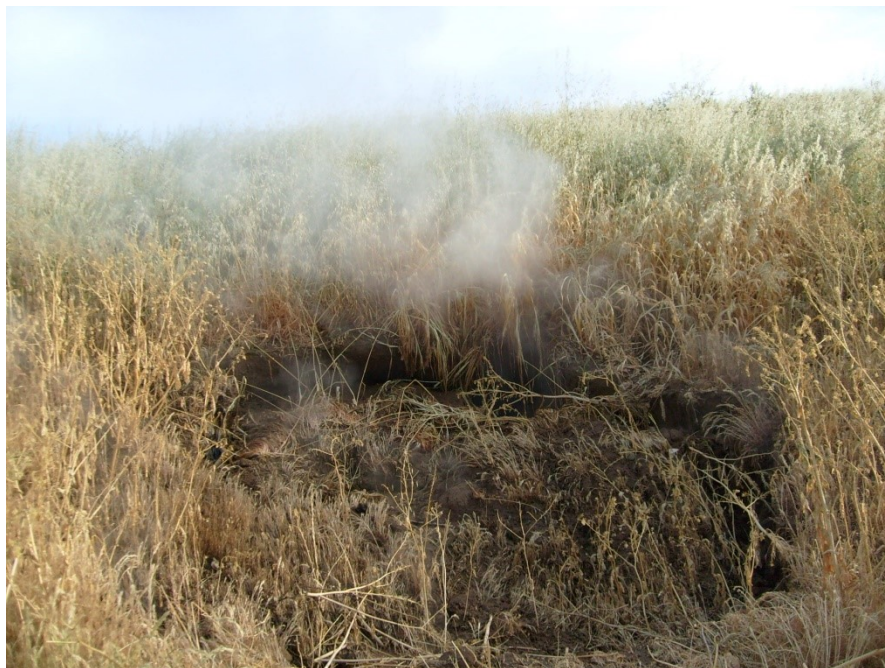
Photo 13. Typical sinkhole at a solid waste landfill caused by a subsurface smoldering event (Source: Todd Thalhamer)
