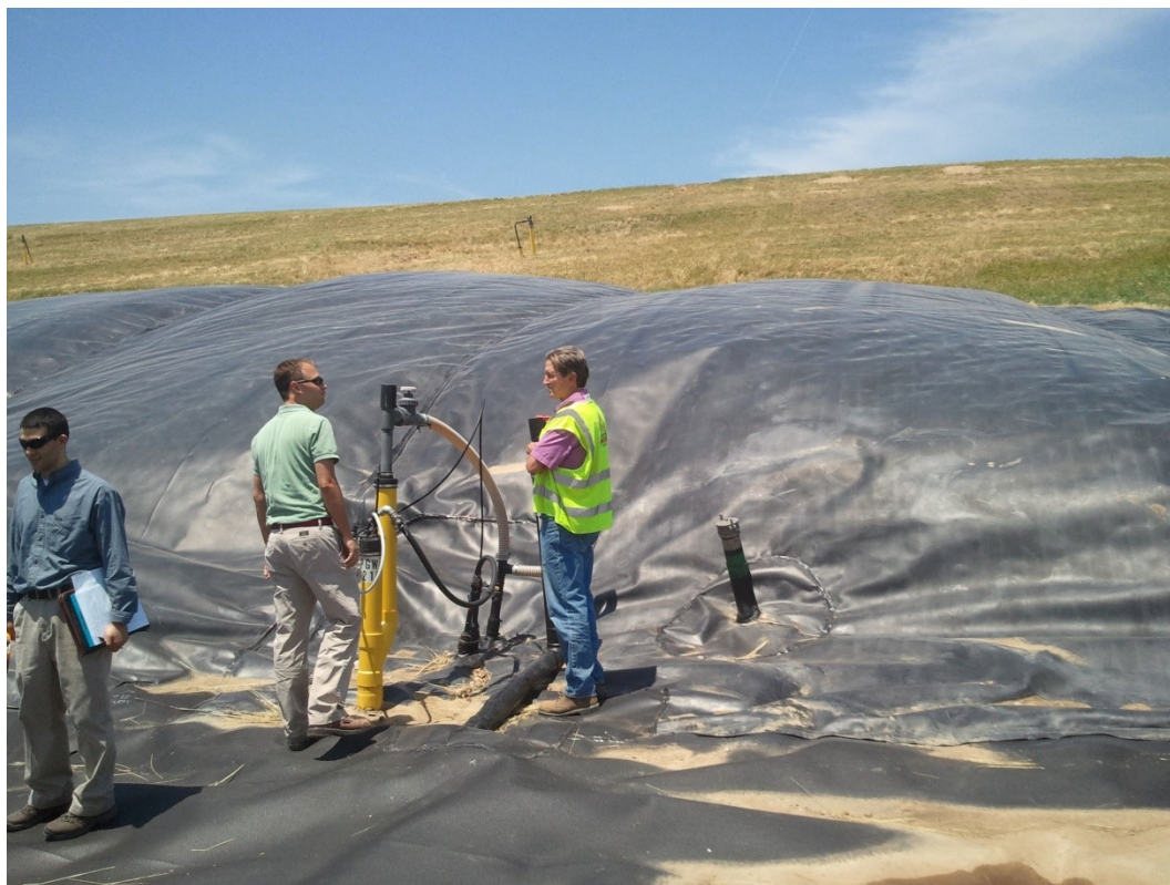
Photo 6. Excessive landfill gas and inflated FML dated June 2012 (Source: Todd Thalhamer 2012).
