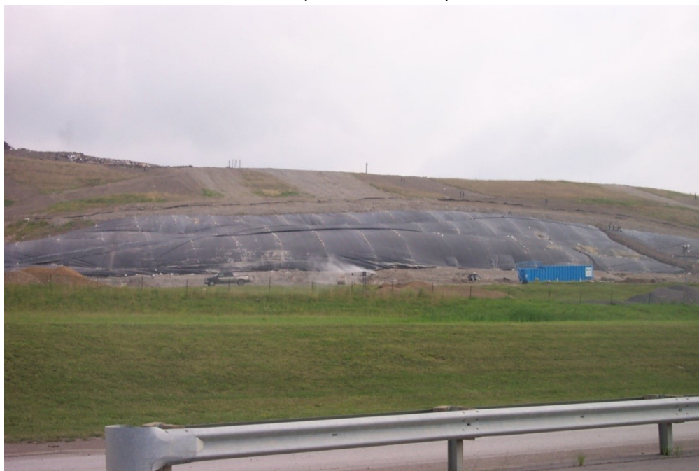
Photo 16. Landfill Gas buildup Under the Geomembrane Cover at Countywide Landfill, Ohio, Summer 2006. (Source: Ohio EPA)
