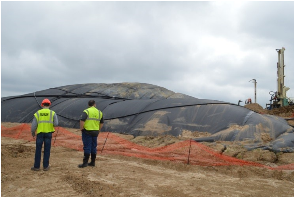
Photo 3. Excessive landfill gas and inflated FML, May 2013 (Source: MDNR Staff, 2013).
