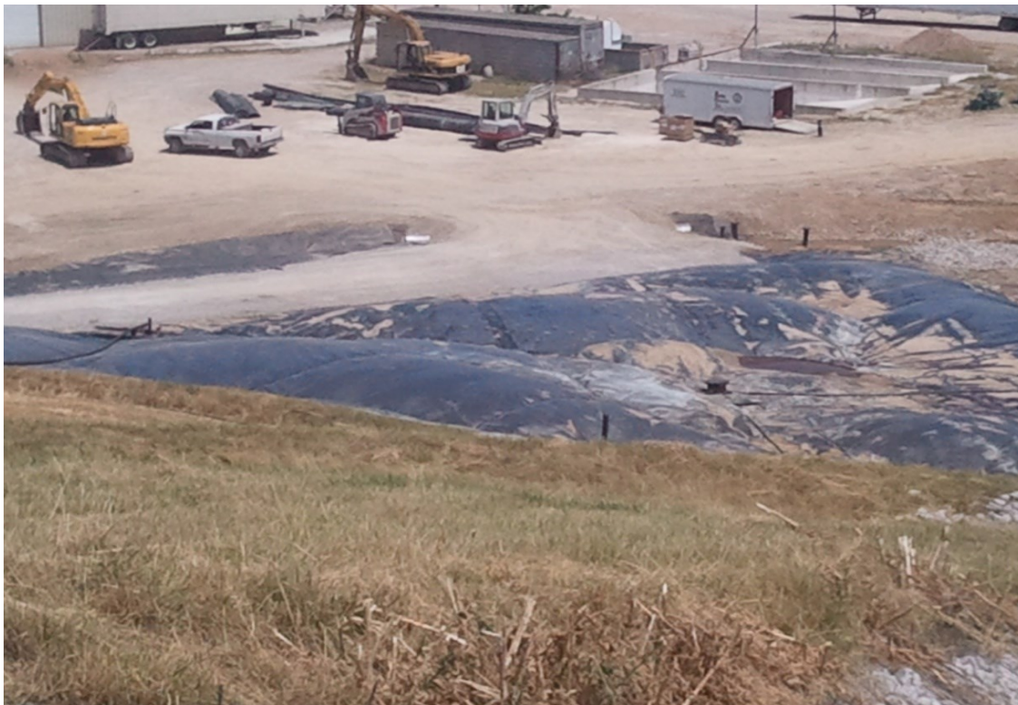
Photo 2: Bridgeton Landfill, St. Louis Area, Missouri, Todd Thalhamer, June 14, 2012. Inflated geomembrane cover in the west bowl settlement area. Significant odors observed.
