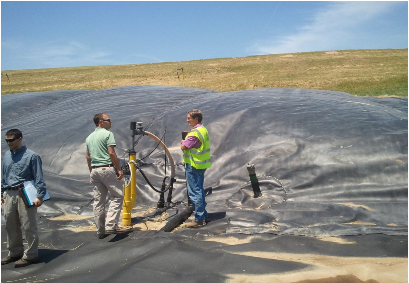
Photo 1: Bridgeton Landfill, St. Louis Area, Missouri, Todd Thalhamer, June 14, 2012. Inflated geomembrane cover in the east bowl settlement area. Significant odors observed.
