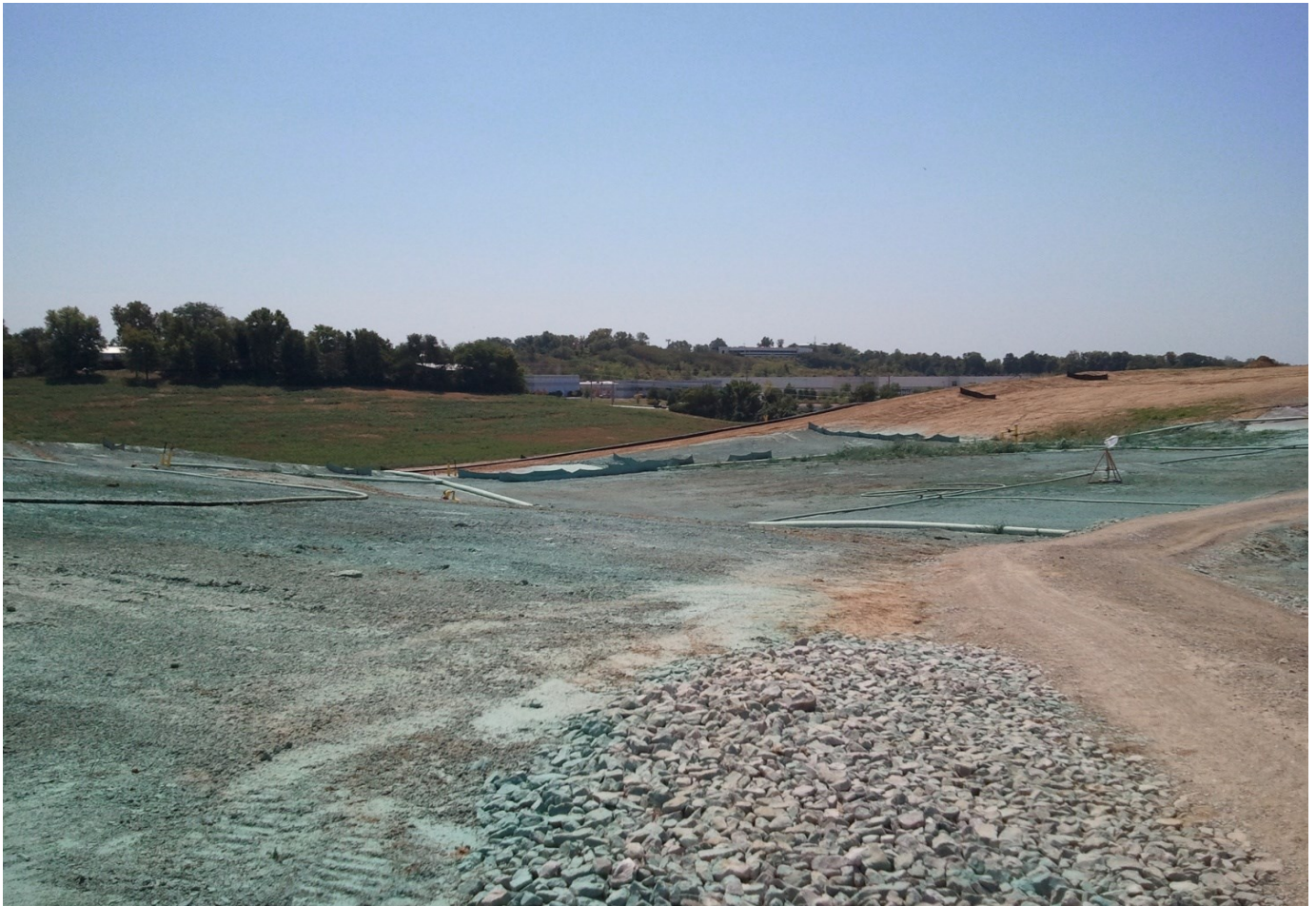
Photo 1: Bridgeton Landfill, St. Louis Area, Missouri, Todd Thalhamer, August 22, 2012. Photos shows the area of the east bowl settlement and additional cover construction.
