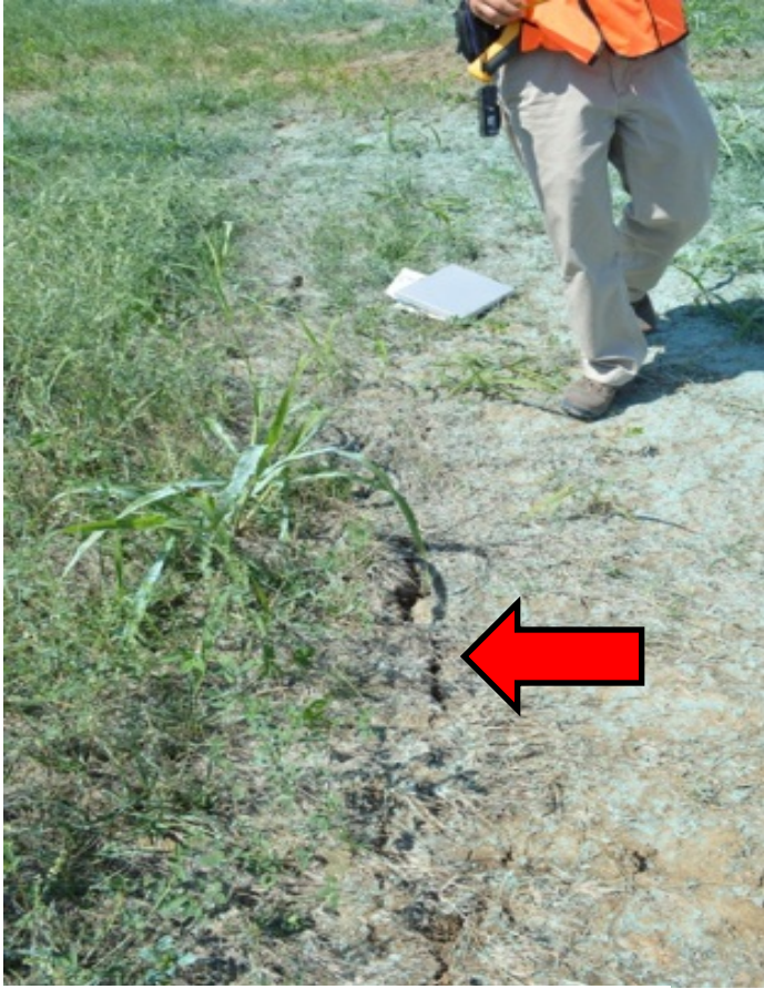
Settlement cracks.
