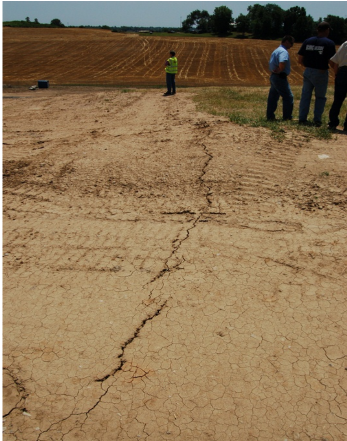
Settlement crack.
