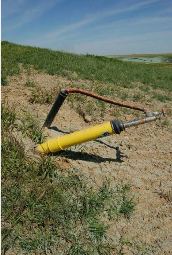
Damaged Gas Collection Well.
